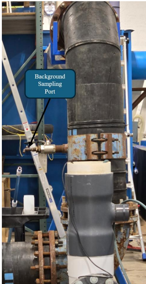
Figure 13 - Background Sampling Port Test Loop 2 and 3
