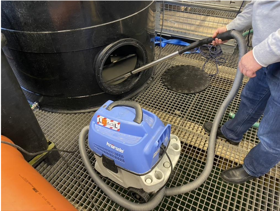
Figure 15 Captured Sediment Collected with Vacuum
