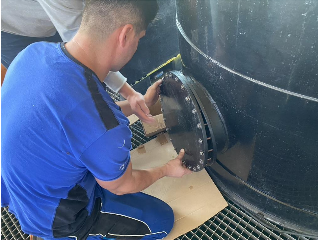
Figure 14 Sediment Sump Removal Port
