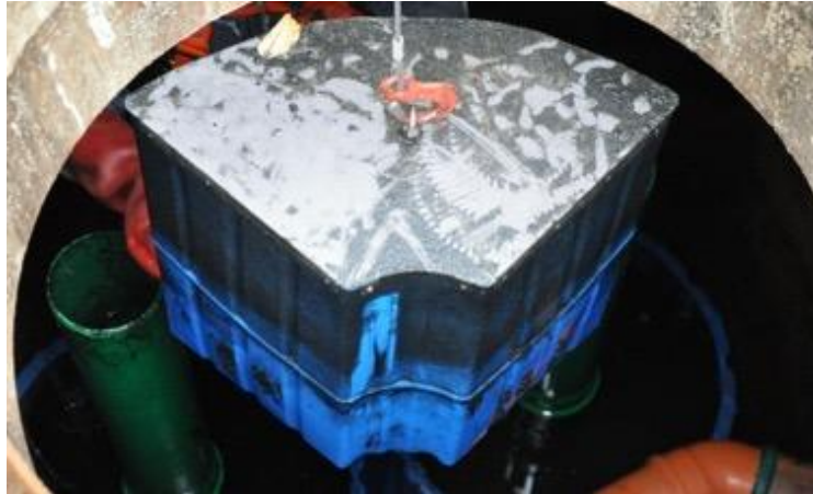
Figure 22 Exchange of a Filter Cartridge
