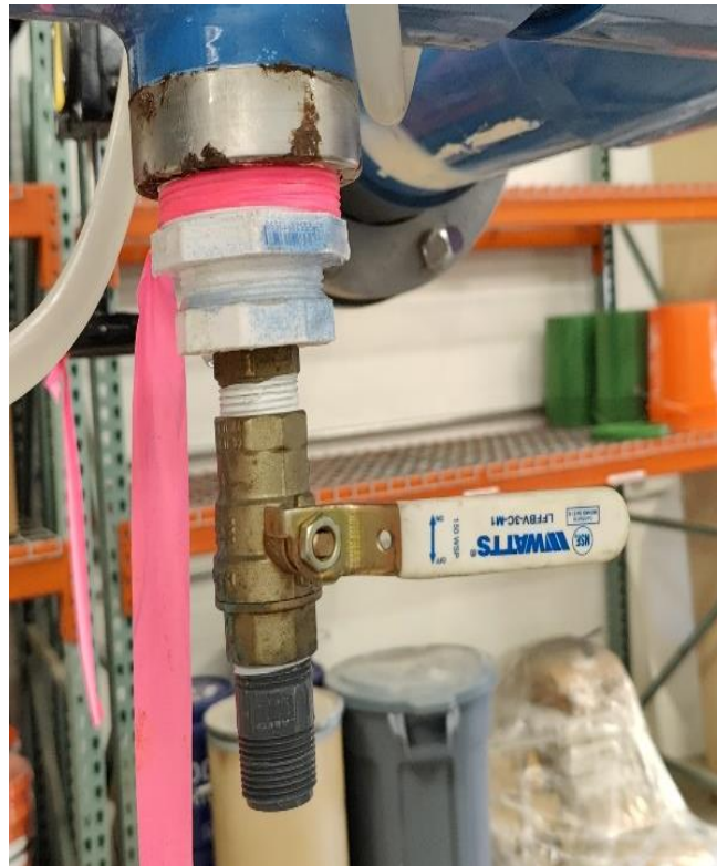
Figure 8 Background Sampling Port
